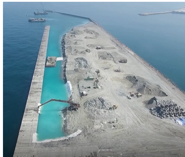
New deep-water berths at Saqr Port
